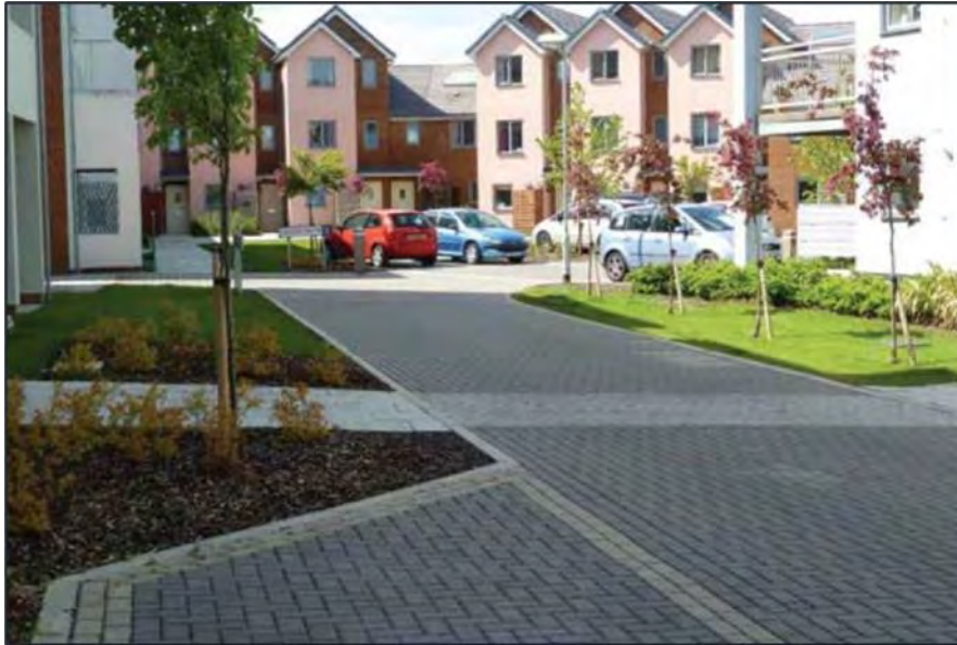
Figure 2 Permeable paving with below ground attenuation (Extract from the SuDS Manual, CIRIA, 2015 [Ref. 9])
